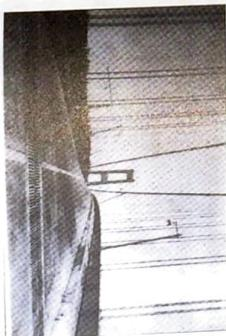
Figure 3.7 The Tacoma Narrows Bridge shortly before its collapse in 1940. The sidewalk to the right is over 28 ft above the one to the left.
