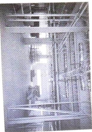
Figure 3.11 Ductwork system with several area changes.
