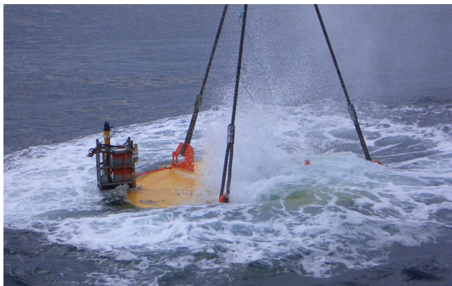
Figure 4-1 Top-plate of suction anchor crossing the water surface. Water spray from ventilation hole.
