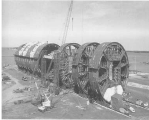
Figure 7.81 Construction of the spar (Technip Offshore)
