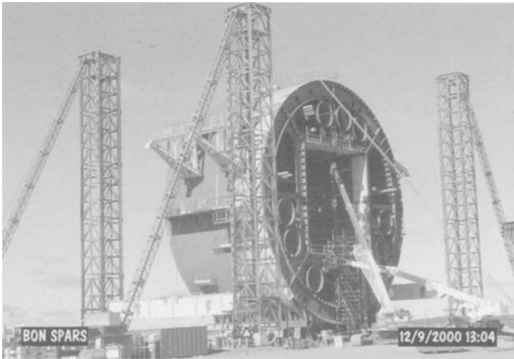
Figure 7.80 Connection of two half-sections (Technip Offshore)
